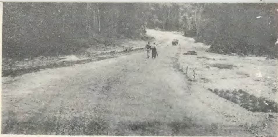
A New Section of the Bartica-Potaro Road.
