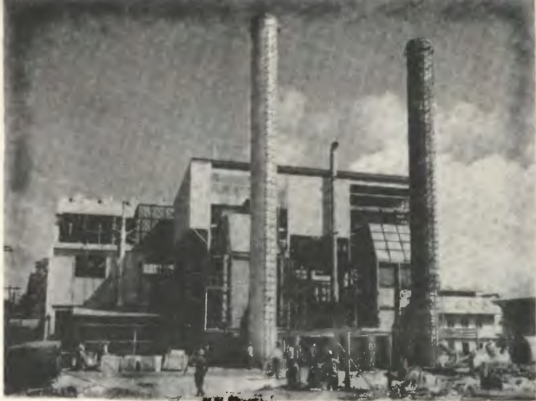
Power Plant of the B.G. Electricity Corporation.
